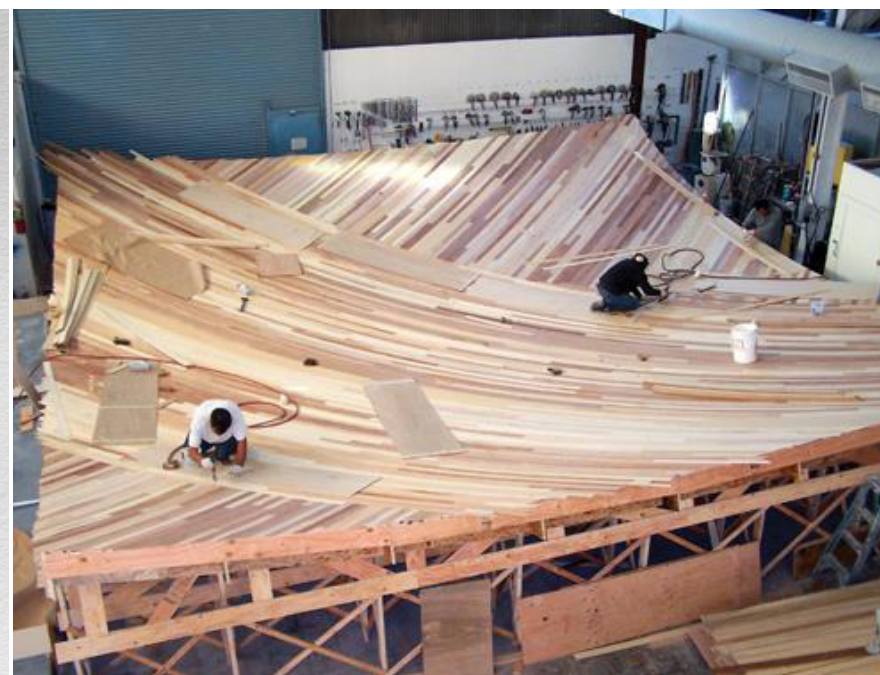
Fabrication and assembly
