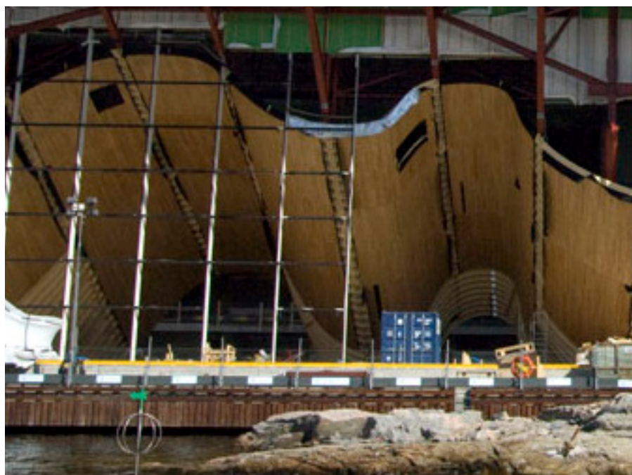
Prefabrication and on-site assembly of timber roof structure
